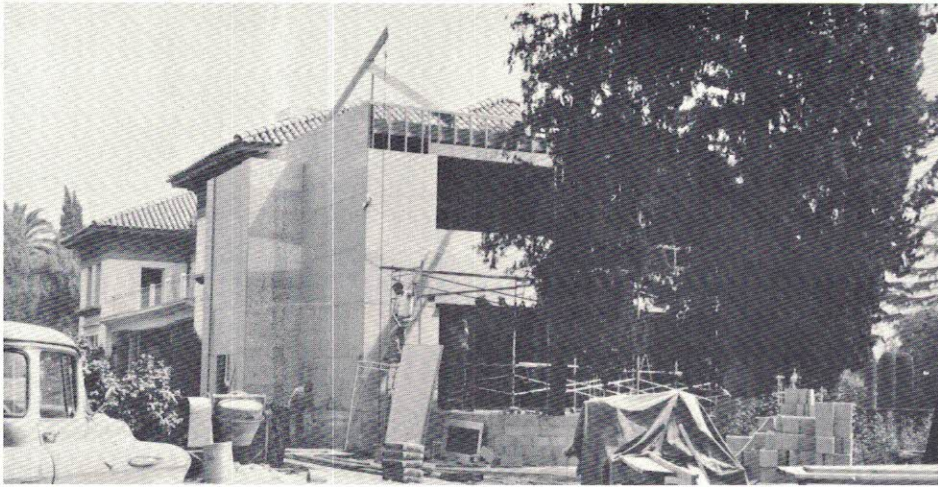
Experimental lab being constructed: new world history classroom.
